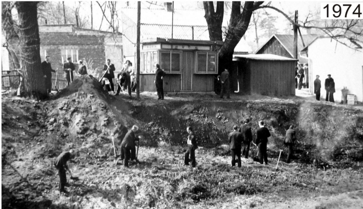
Fig. 2: Anthropogenic changes of Kamionka riverbed in 1974 under construction of Suchedniów Lake (Piasta 2012)
